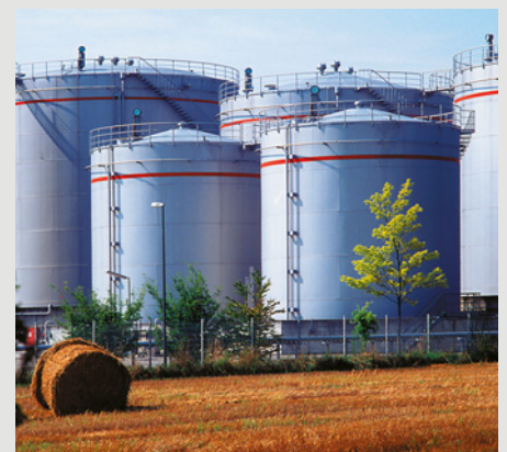
Industrial steel constructions
